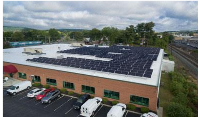
Ryan Insurance's building on Ulster Avenue showing the white reflective roof and bifacial solar panels.
